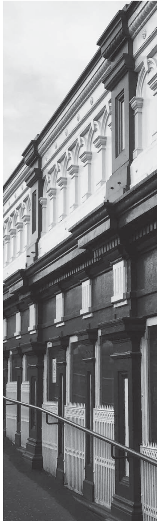
Ductile Iron Parapets for Waverley Station cast by Ballantine Castings
