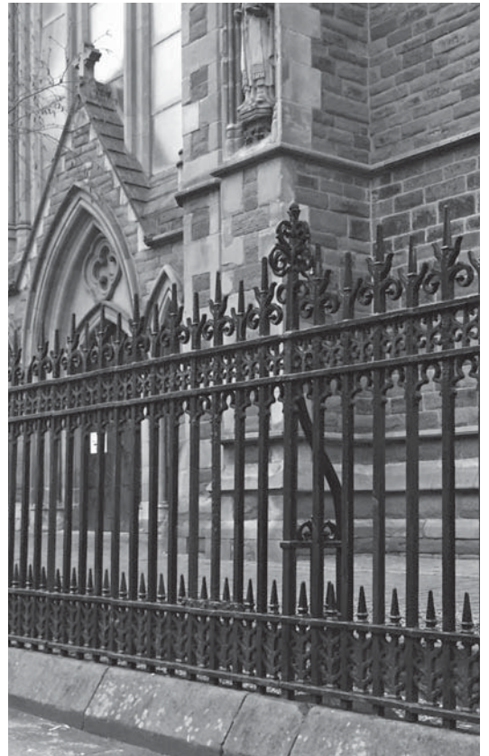
Church railing refurbishment in cast iron by Ballantine Castings
