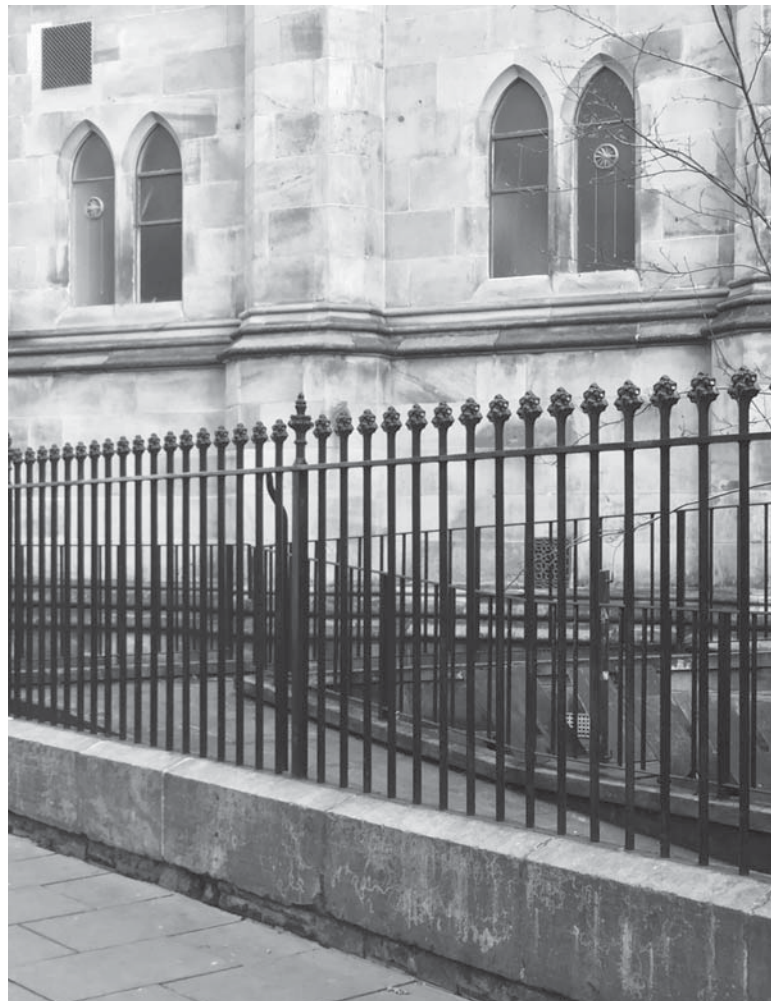
Ductile iron railings supplied by Ballantine Castings which we designed from an old photograph
